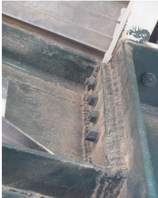
Figure II. 5: Assemblage poteau-poutre
