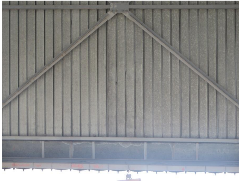
Figure II. 9: Les diagonales de contreventement horizontal
