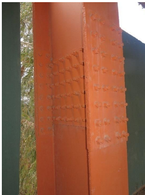
Figure II. 6: Assemblage poteau-poteau
