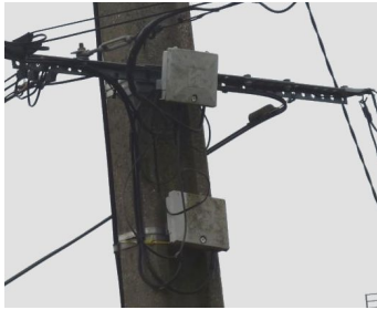
FIGURE 12 – Point de concentration
