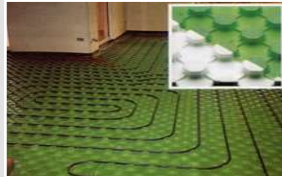
Plancher chauffant
